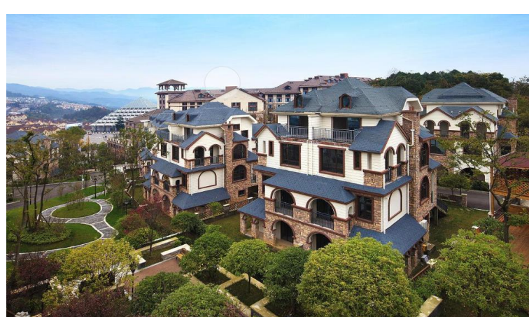
Villa area emergency power
